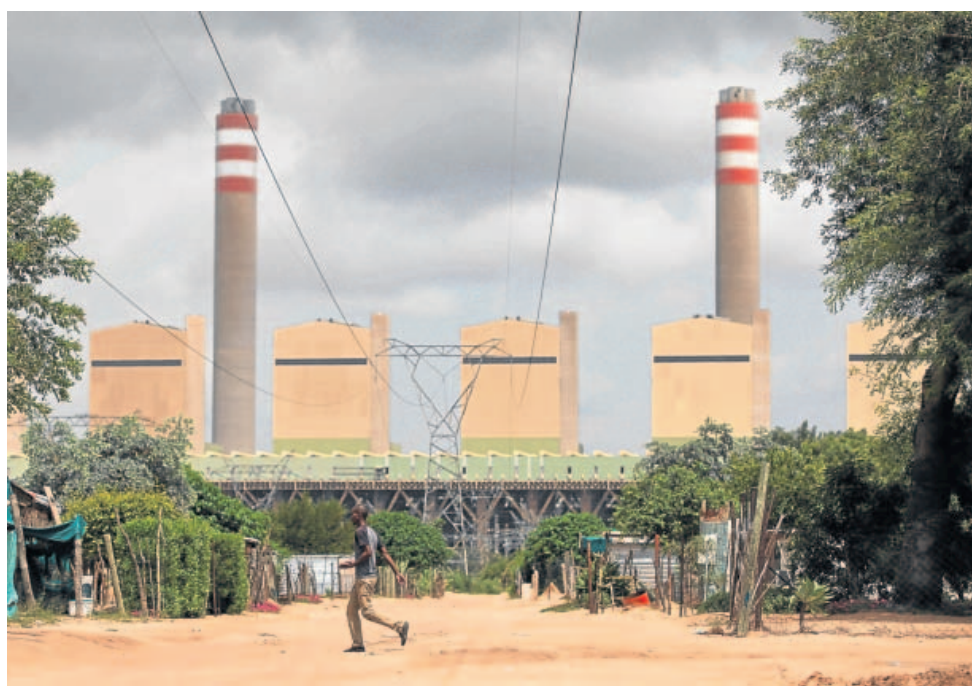
The total system stockpile for all power stations is 67 days. / Alastair Russell
